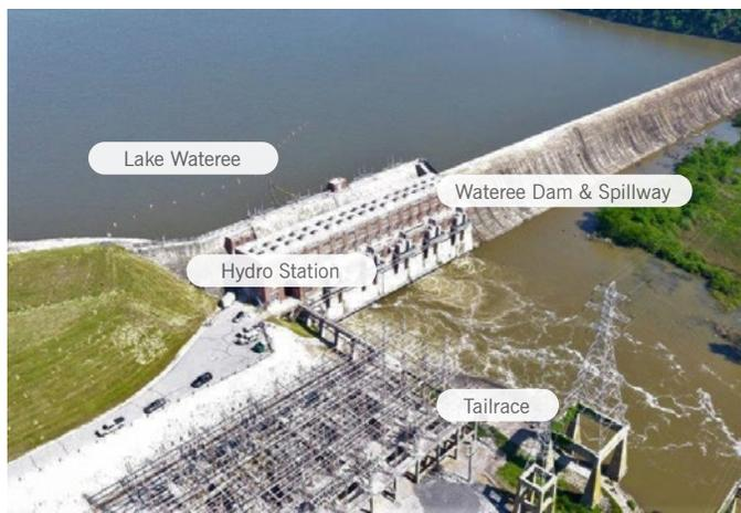
The Wateree spillway is an overflow spillway, which means it does not have flood gates that can be opened to release water during high inflow events. The installation of Obermeyer gates will provide a way to release more water in a controlled manner from the lake. This will help reduce the frequency and degree of small to moderate flooding events.
